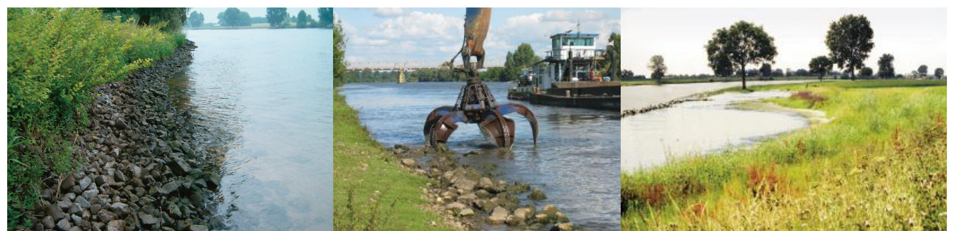
Constructing free eroding banks as a landscaping measure.
