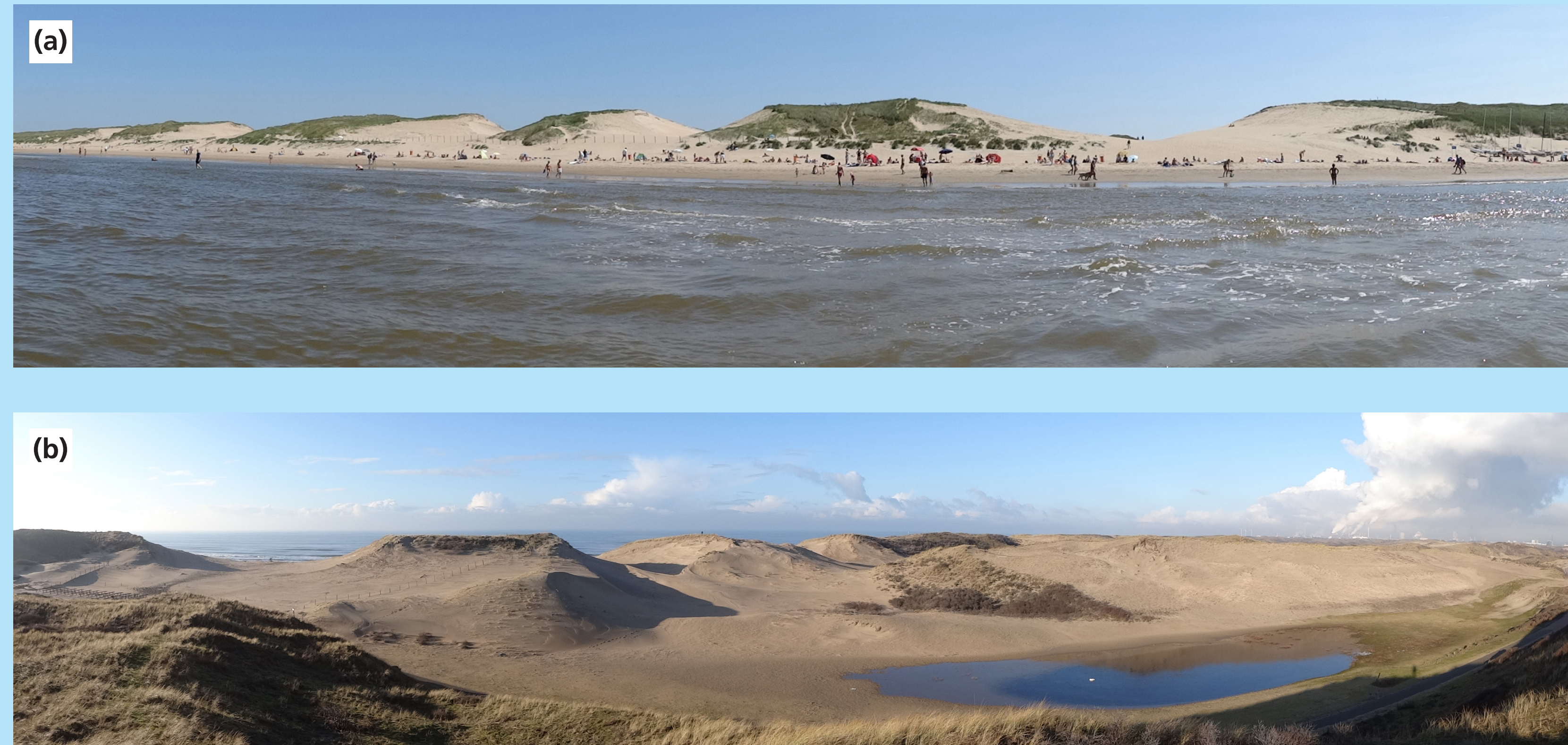
Figure 1 Man-made notches through the 20-m high foredune at National Park Zuid-Kennemerland (Netherlands) viewed (a) from the sea and (b) an inland dune. The notches were dug in the 2012/2013 winter. In total, about 180,000 m 3 of sand was removed. The initial width of the notches was 50-100 m, their cross-dune length was 60-120 m, and the highest part of the notch floor was 9 m above Mean Sea Level.
