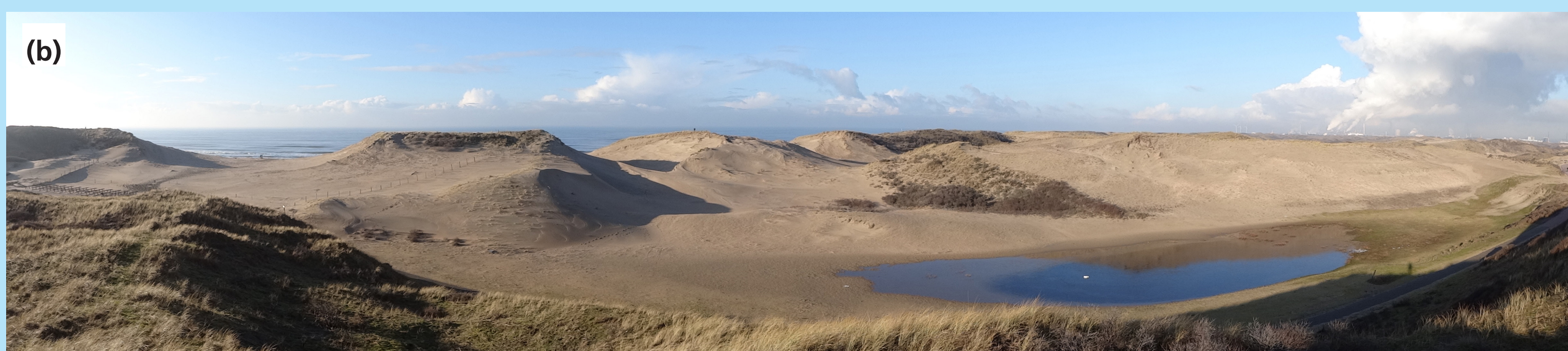
Figure 1 Man-made notches through the 20-m high foredune at National Park Zuid-Kennemerland (Netherlands) viewed (a) from the sea and (b) an inland dune. The notches were dug in the 2012/2013 winter. In total, about 180,000 m 3 of sand was removed. The initial width of the notches was 50-100 m, their cross-dune length was 60-120 m, and the highest part of the notch floor was 9 m above Mean Sea Level.
