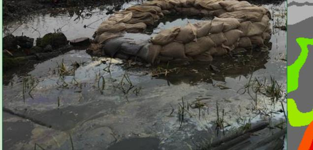
Piping is the creation of a subsurface pipe as a result of seepage induced erosion (usually during high water events). This process can be approached from different scales. On the **delta scale** general delta wide trends can be used to predict general piping conditions. On the **regional scale** the position and orientation of individual channel belts precondition piping potential. At the process scale small scale subsurface variations determine if **piping is able to progress.**
